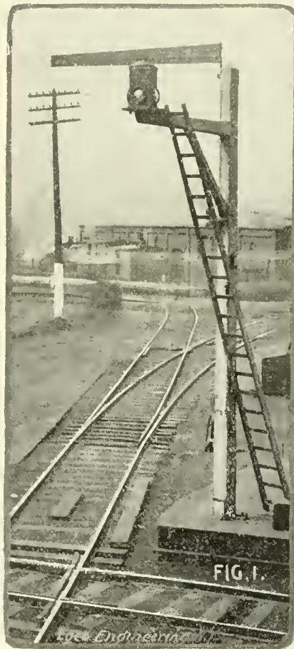
A SIMPLE CROSSING SIGNAL.
